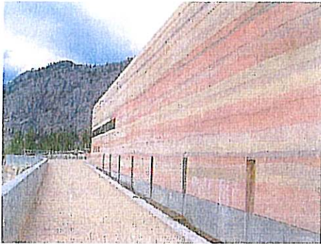
Figure 2: Example of rammed-earth wall at Nk'Mip Desert Cultural Centre
